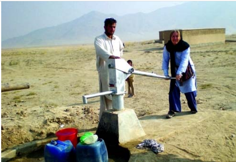
Pumped up. Traylor Kulshan tests a new well north of Kabul, Afghanistan.
